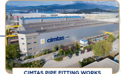
ÇİMTAŞ PIPE FITTING WORKS
