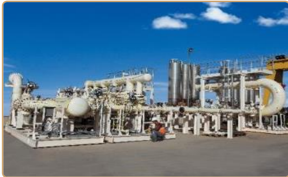
Rominserv Storage Tanks Farm Revamping Romania, EMERSON-DANIEL
