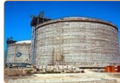
2 x 140,000 m 3 EGEGAZ LNG, Tank Farm, Turkey, EGEGAZ
