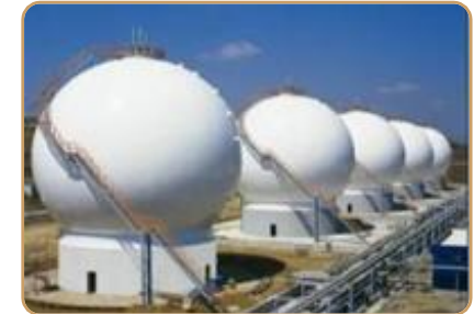
Spherical Storage Tanks, Marmara Ereğlisi, BUTANGAZ
