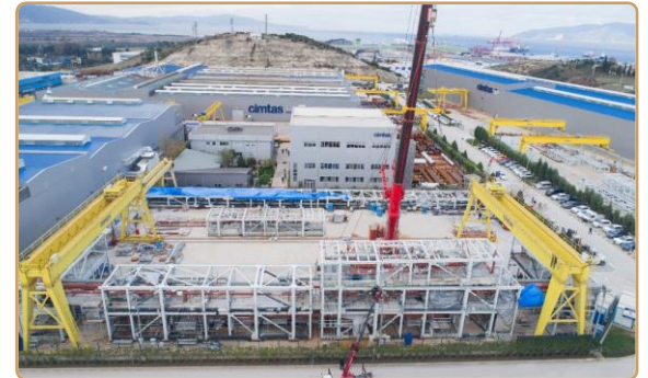
Piping Modularization, EVM II CCPP, Mexico, GE Power
