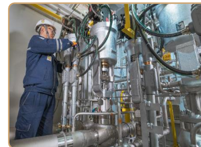
Fuel Gas Skid, MHPS
