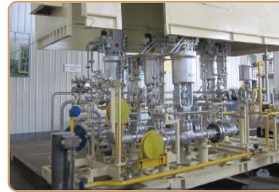
Fuel Gas Skid, GE
