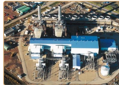
790 MW, Rijnmond Energy Center, the Netherlands, BECHTEL-ENKA JV
