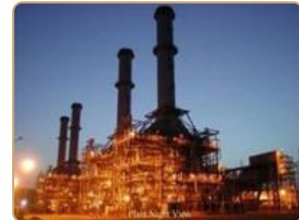
1,532 MW, Izmir CCPP, Turkey, ENKA
