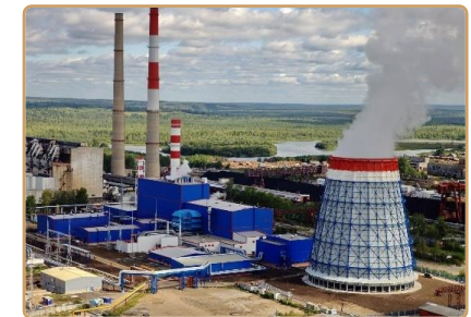
411 MW, Yajva CCPP, the Russian Federation, ENKA
