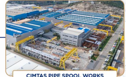
ÇİMTAŞ PIPE SPOOL WORKS
